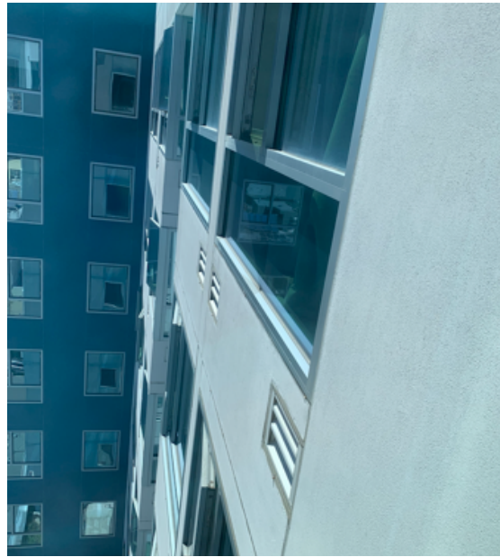
Windows at 10 th Floor
