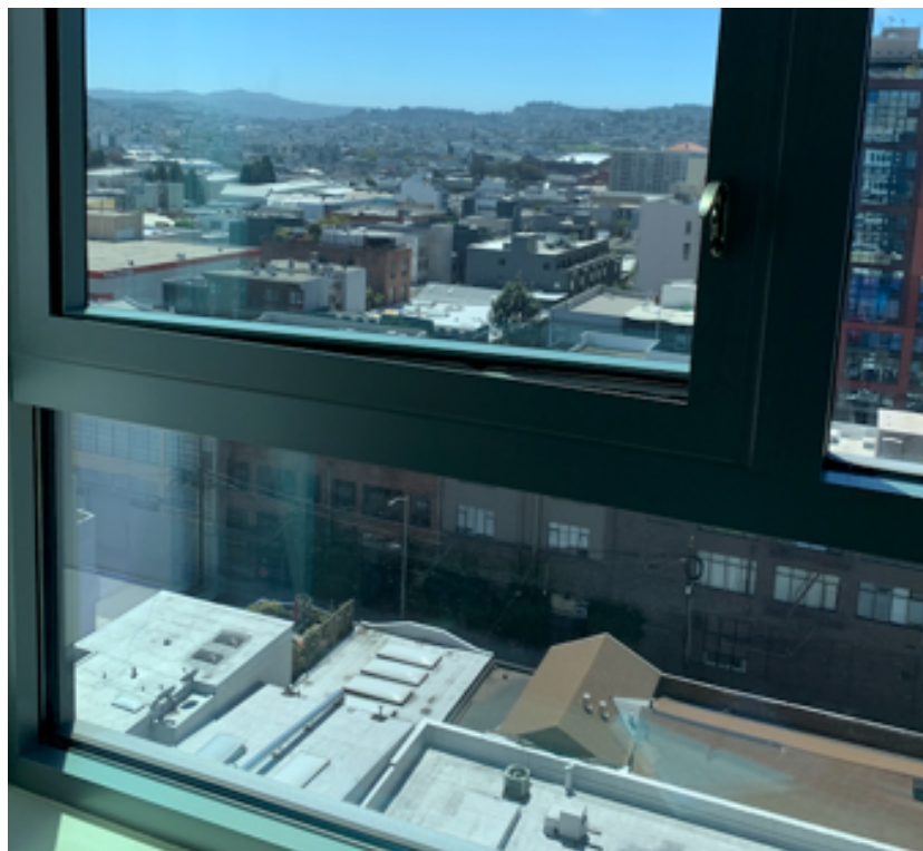
Casement and fixed paned windows in apartment unit
