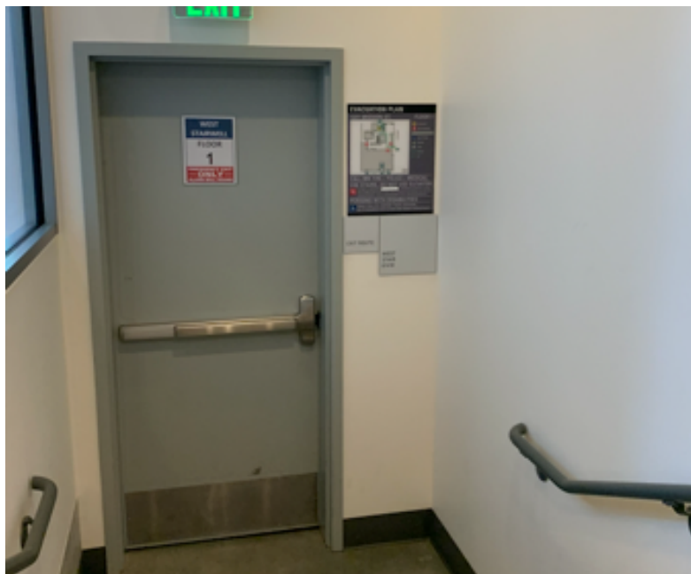
Exit door (west) and evacuation signage. This door leads to Washburn Alley.
