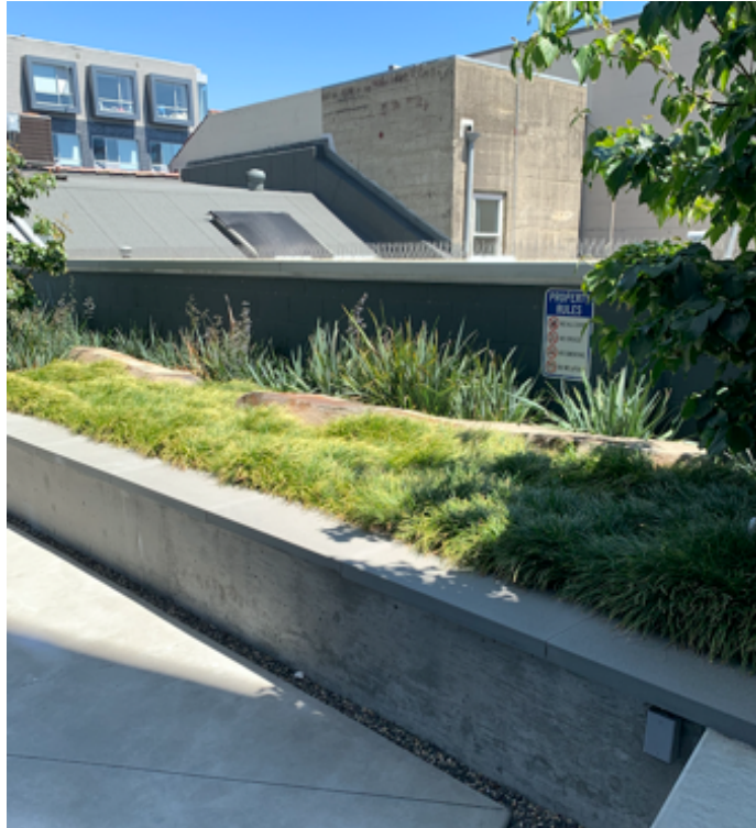
Second floor courtyard planted area
