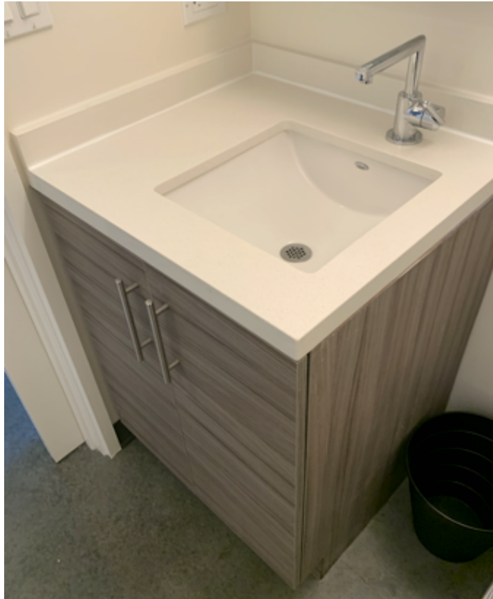
Typical bathroom sink and cabinet
