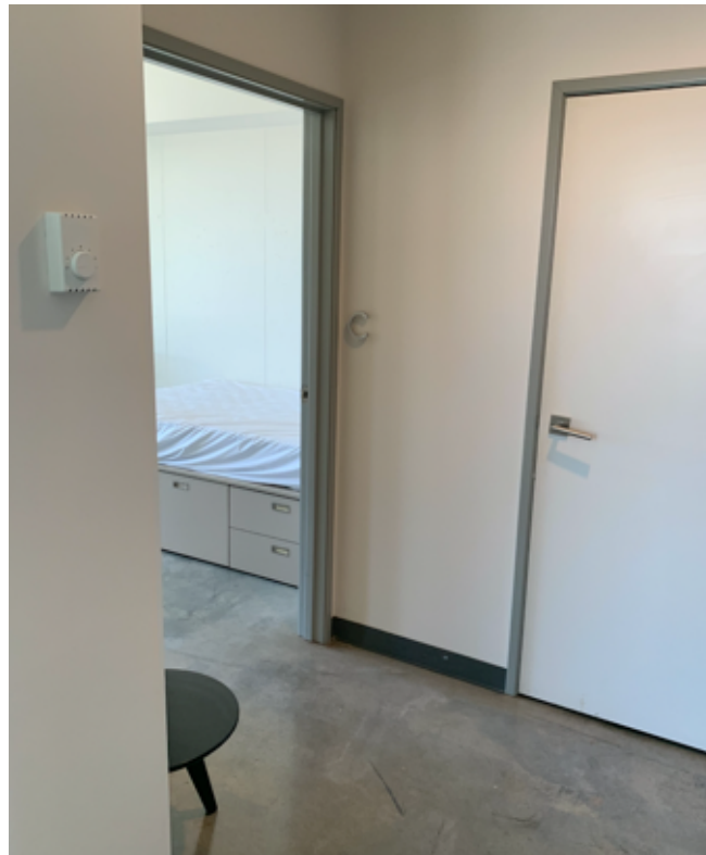
Flooring in three-bedroom suite hallway
