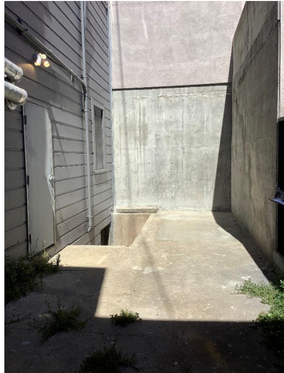
Rear Patio, Stair to Basement, and Door to Residential Stair
