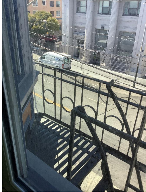
Window and Fire Escape
