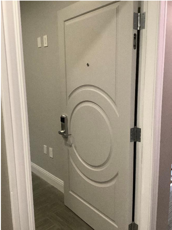
Unit Entry Door with Card Reader
