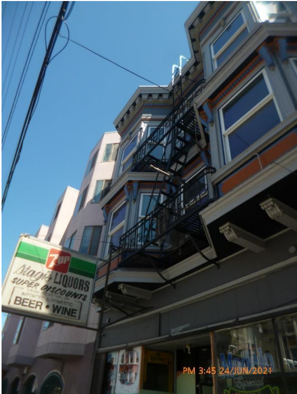
Building Front Façade
