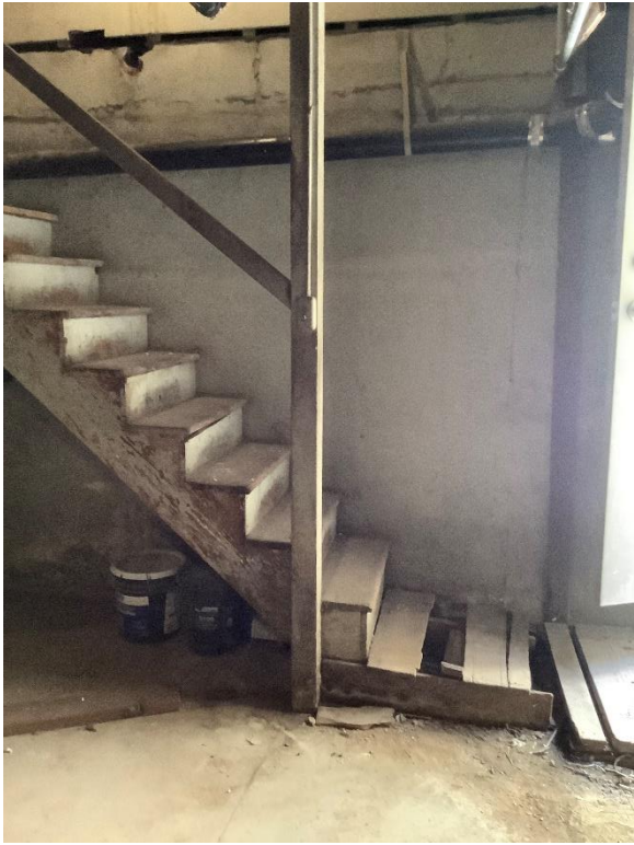
Basement Wooden Staircase
