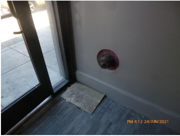
Residential Vestibule and Existing FDC
