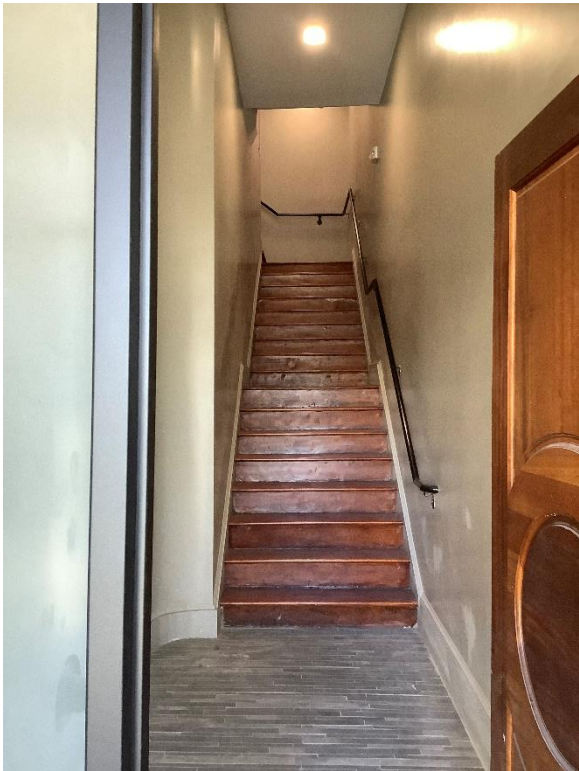
Residential Vestibule and Exit Stairs
