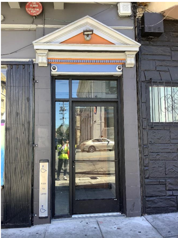
Residential Entrance, Hi-Lo Door Actuator, Lighting
