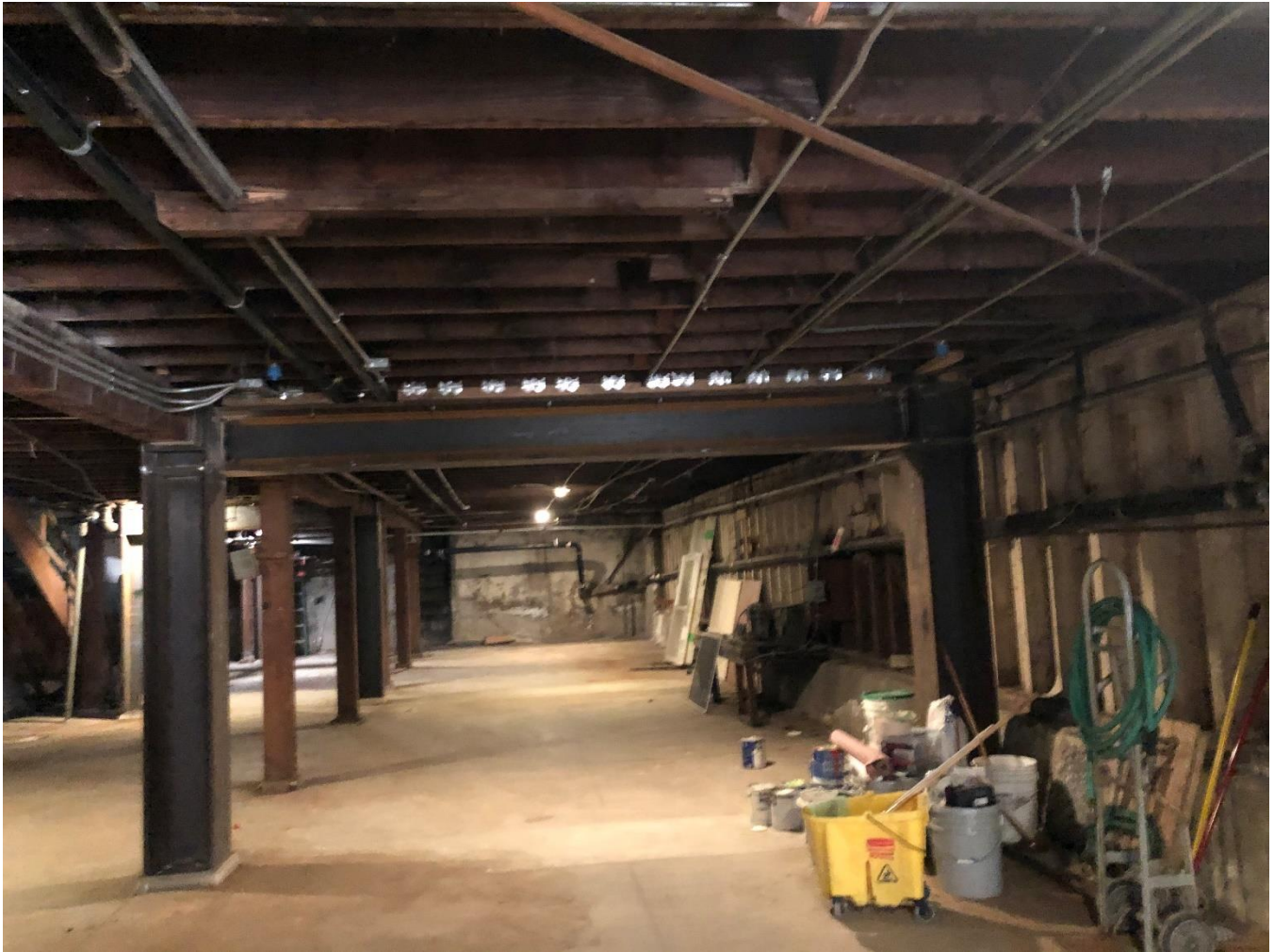
Photo 3. Moment frame in the basement
