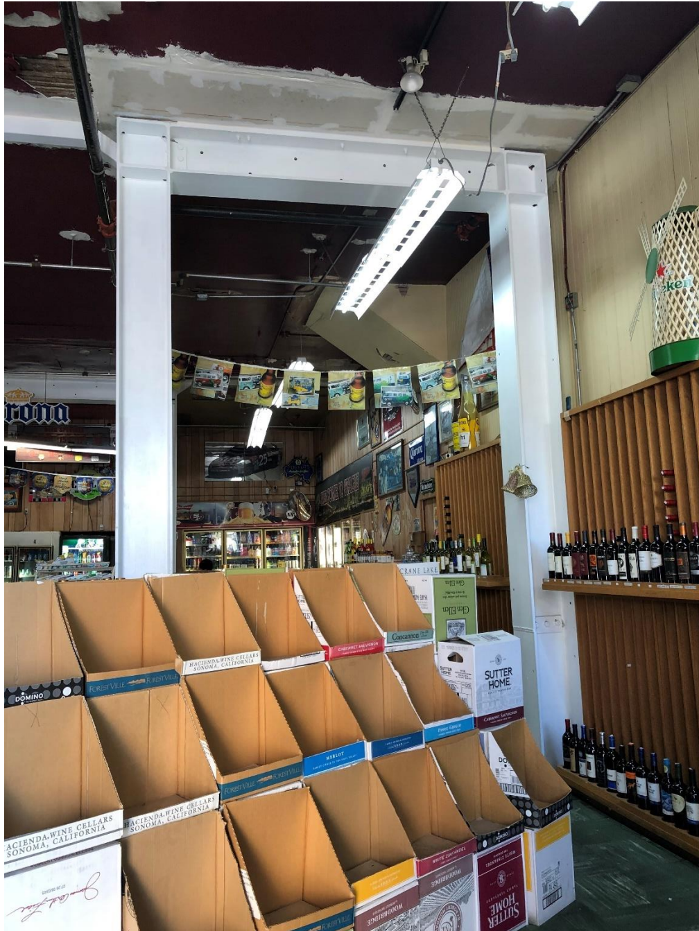
Photo 2. Moment frame in the ground floor commercial space
