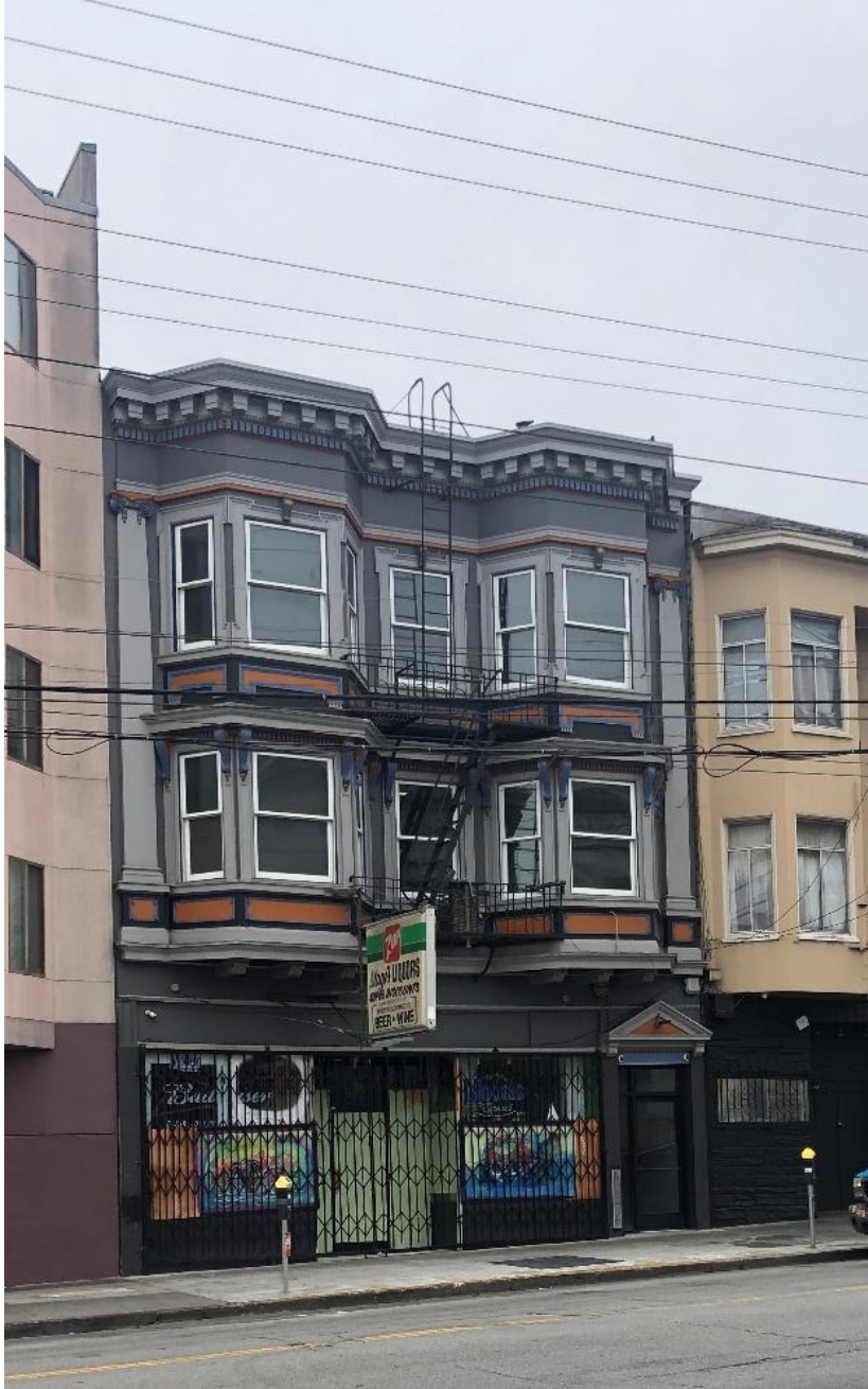
Photo 1. Exterior of building
