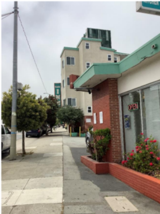
Management Building at public right of way, "tower" part of motel behind.
