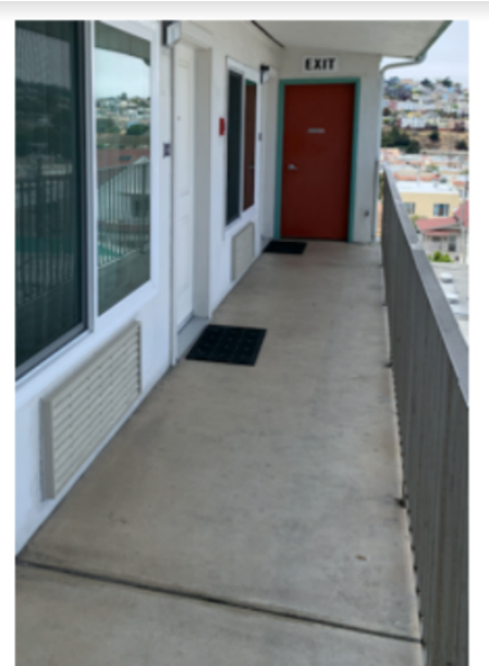
Walkway at 4 th floor of Building A
