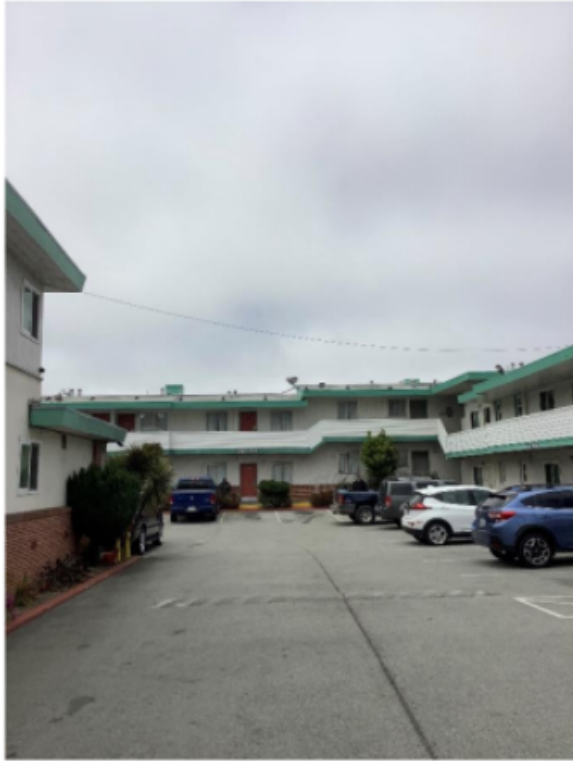
Two-story motel wings, Management Building, Parking Lot
