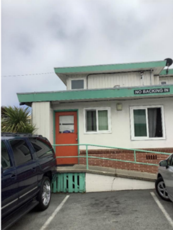
Management Building Rear Exit, Ramp
