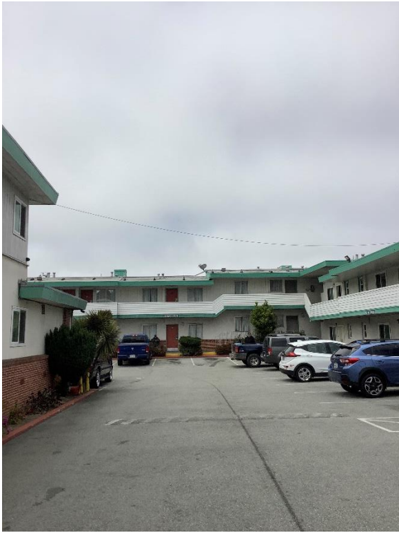
Two-story motel wings, Management Building, Parking Lot
