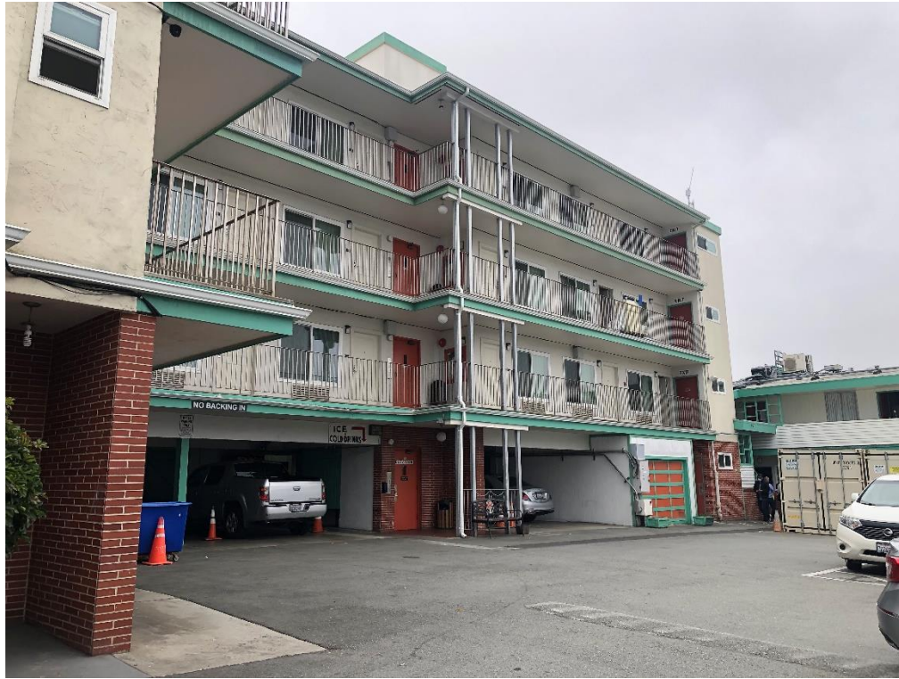
Photo 1. Exterior of Building A
