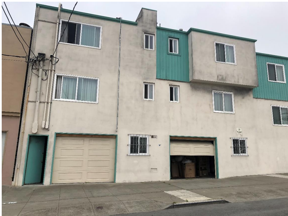
Photo 2. Exterior of Building B from Ellington Avenue
