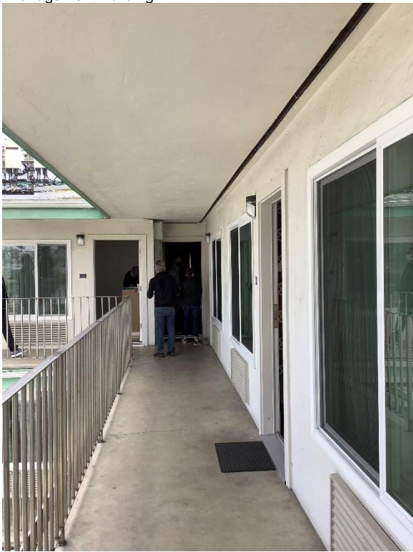
"Tower" exit balcony and guardrail, typical
