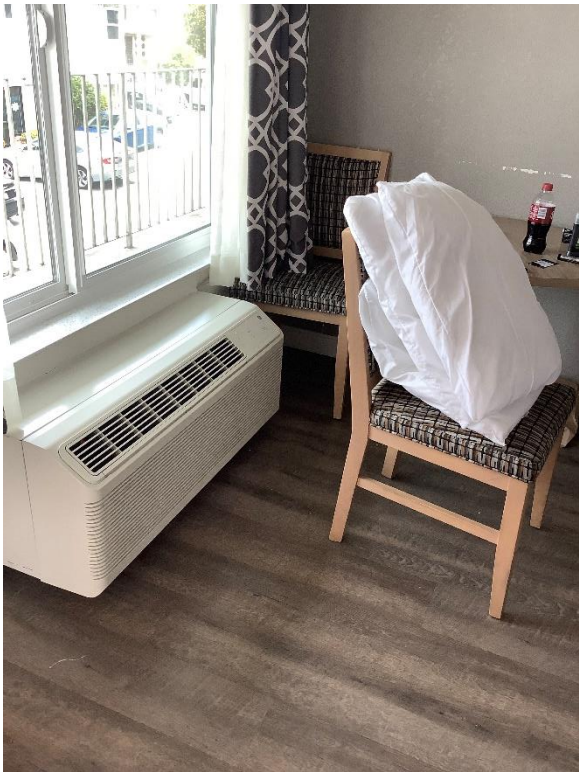
Window Covering, PTAC Unit in renovated motel room
