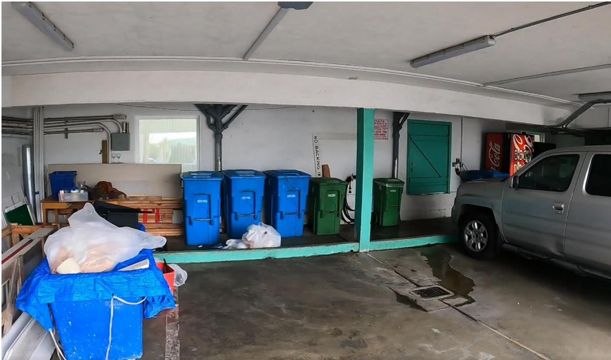
Utility Area, Carport, Trash Collection Area
