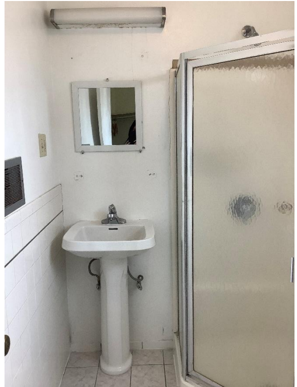
Bathroom in non-renovated motel room
