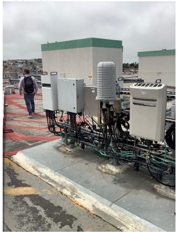
Roof Equipment on "Tower" part of motel
