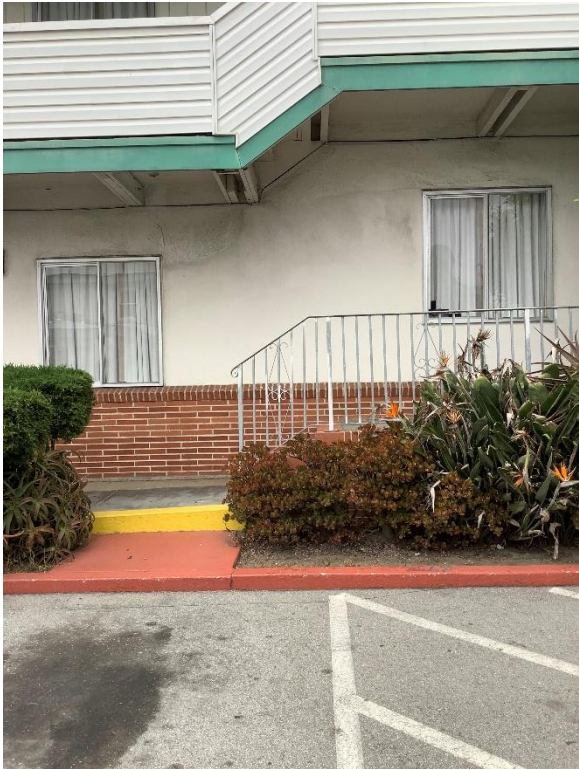
In grade planting, Sloped Walkway to stairs with Guardrail
