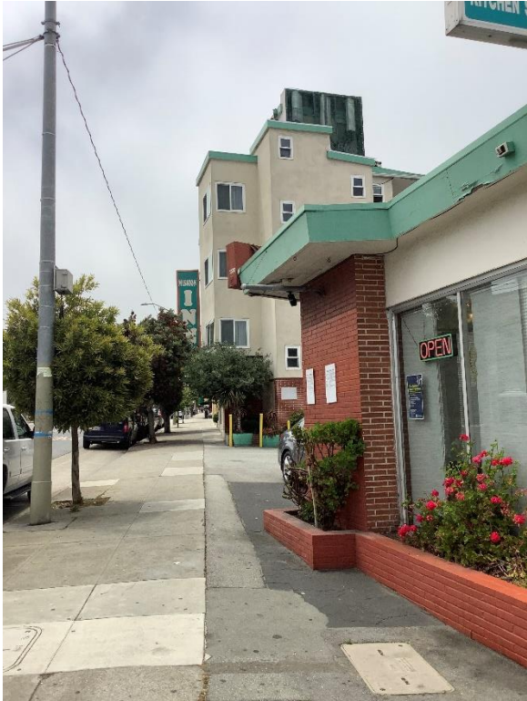
Management Building at public right of way, "tower" part of motel behind.
