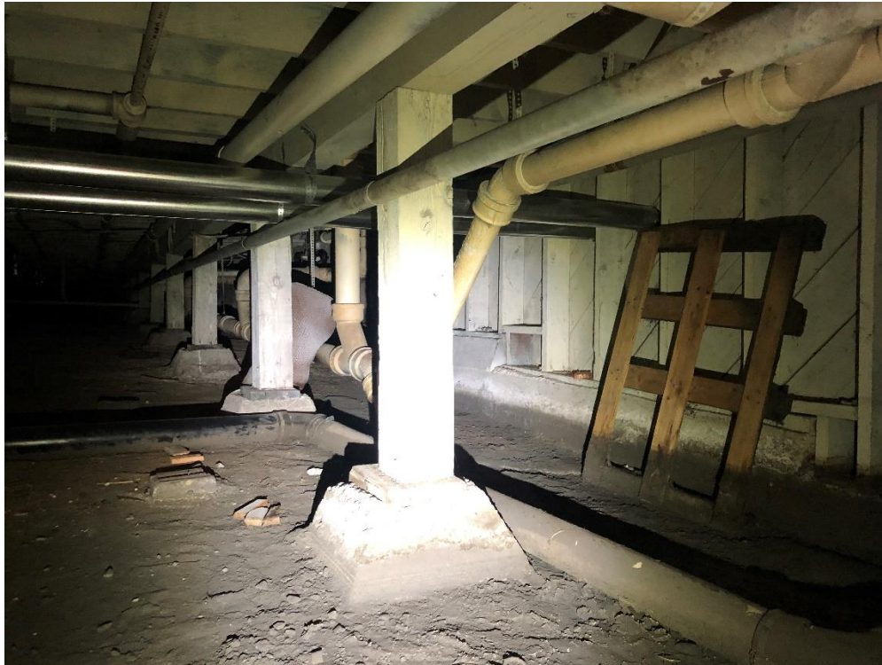
Photo 3. Crawl space under Building B
