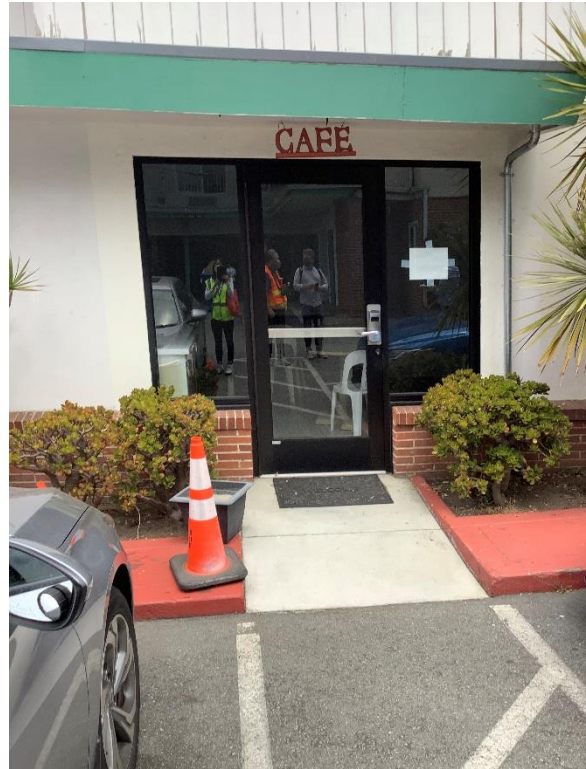
Sloped Walkway to Breakfast Room
