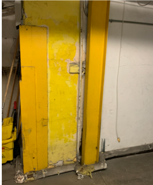
Structural steel at driveway entrance
