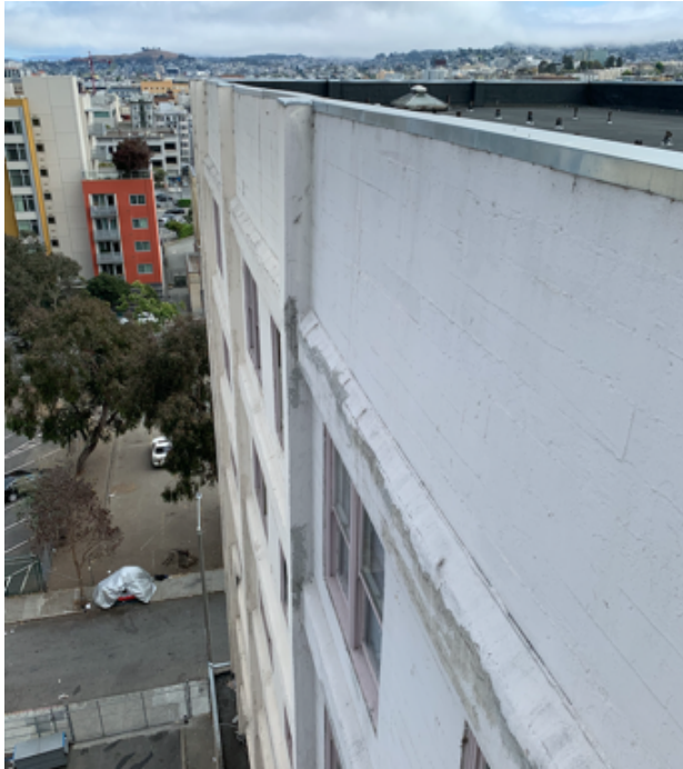
Concrete wall siding at east side of building
