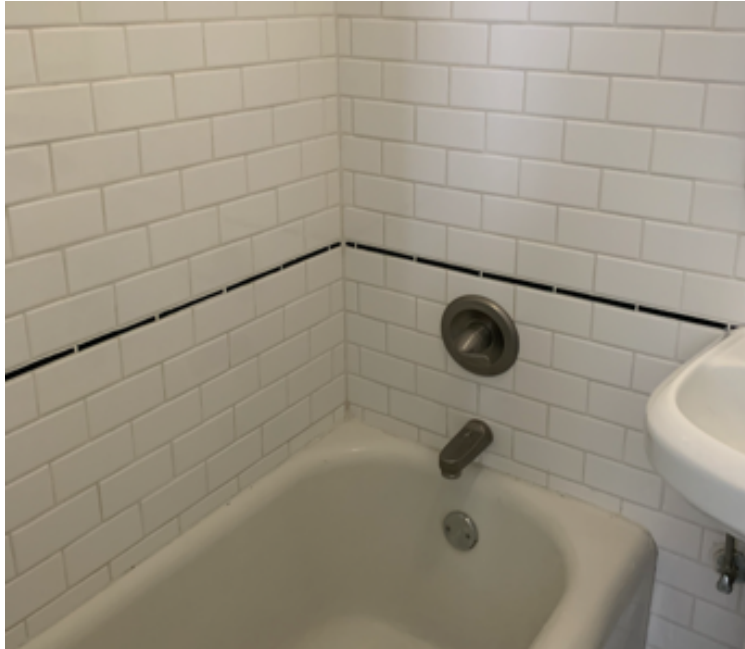
Tub, surround and valve
