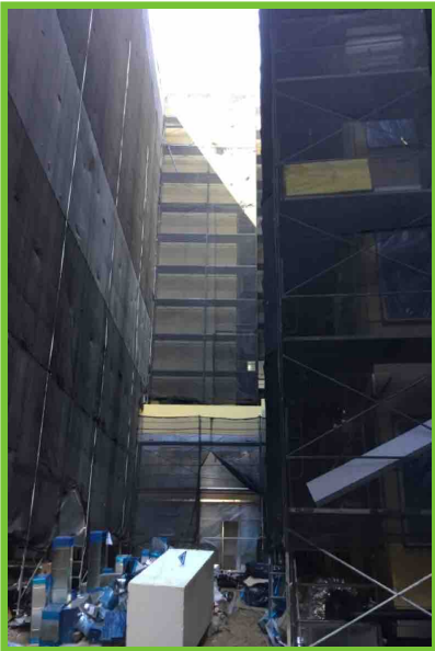
Note: Courtyard west elevation
