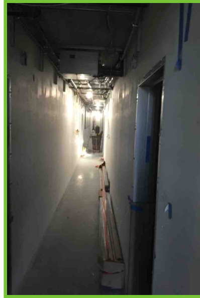
Note: 7th floor corridor B
