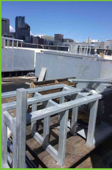
Note: Rooftop planters
