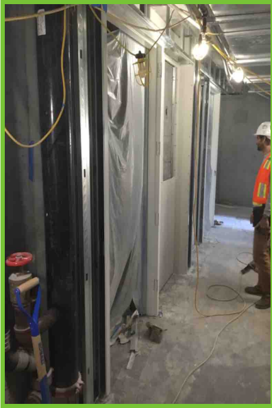
Note: Garden level elevators
