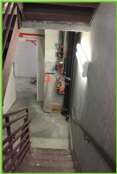
Note: Corridor stairwell 5B
