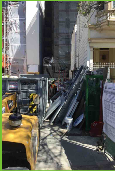
Note: East Facade
