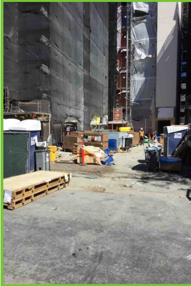
Note: East facade
