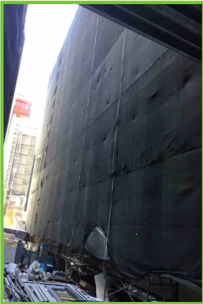
Note: Courtyard covered scaffolding
