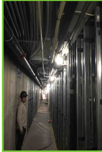
Note: Level G corridor
