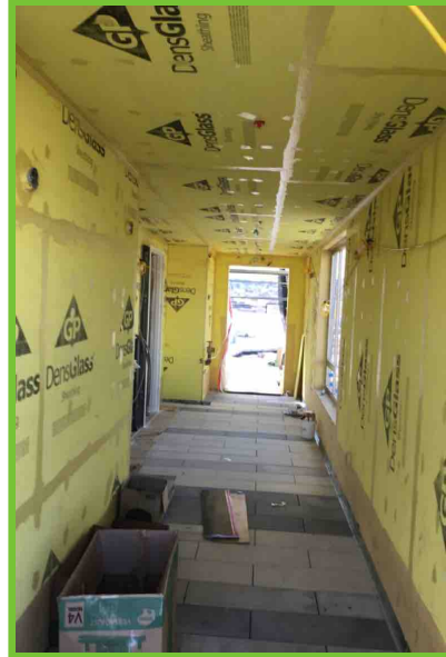
Note: Rooftop elevator lobby
