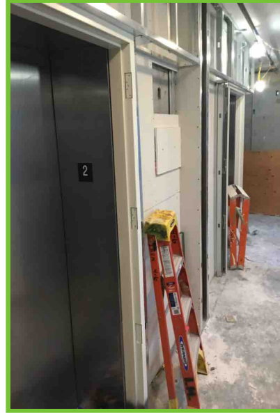
Note: Elevators facing East courtyard
