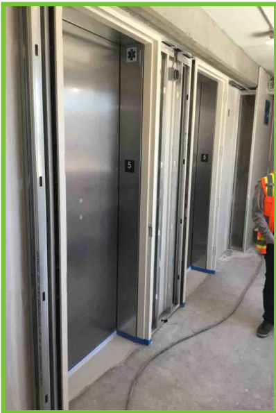
Note: 4th floor west elevators
