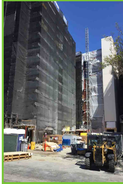
Note: East Facade
