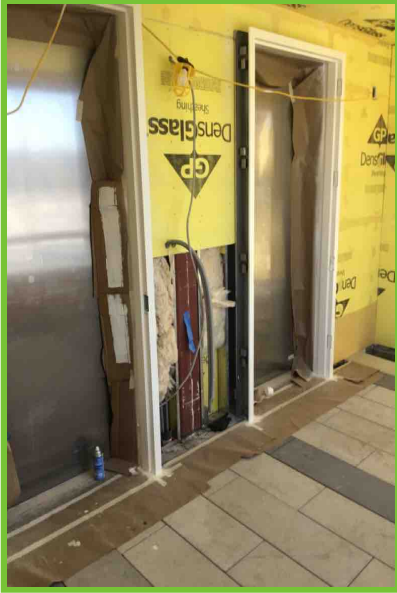
Note: Rooftop elevators
