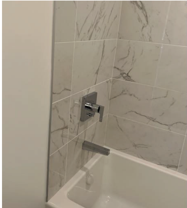
Tile tub surround and fiberglass tub
