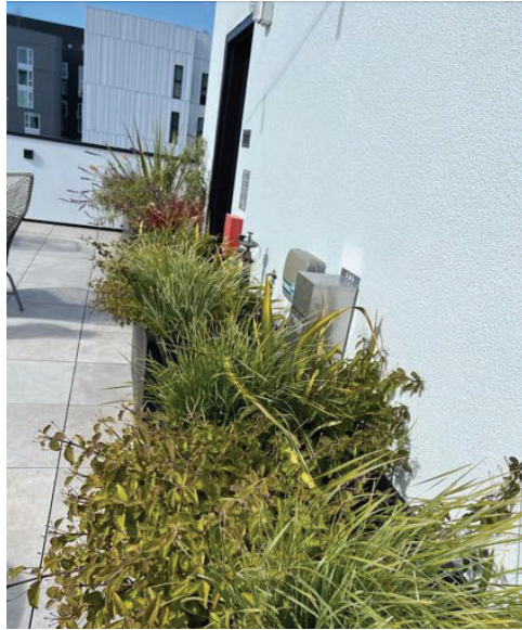
Roof deck planter
