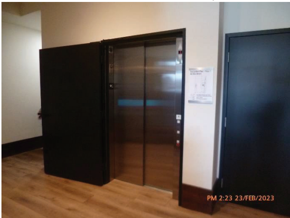
Elevator at the Lobby
